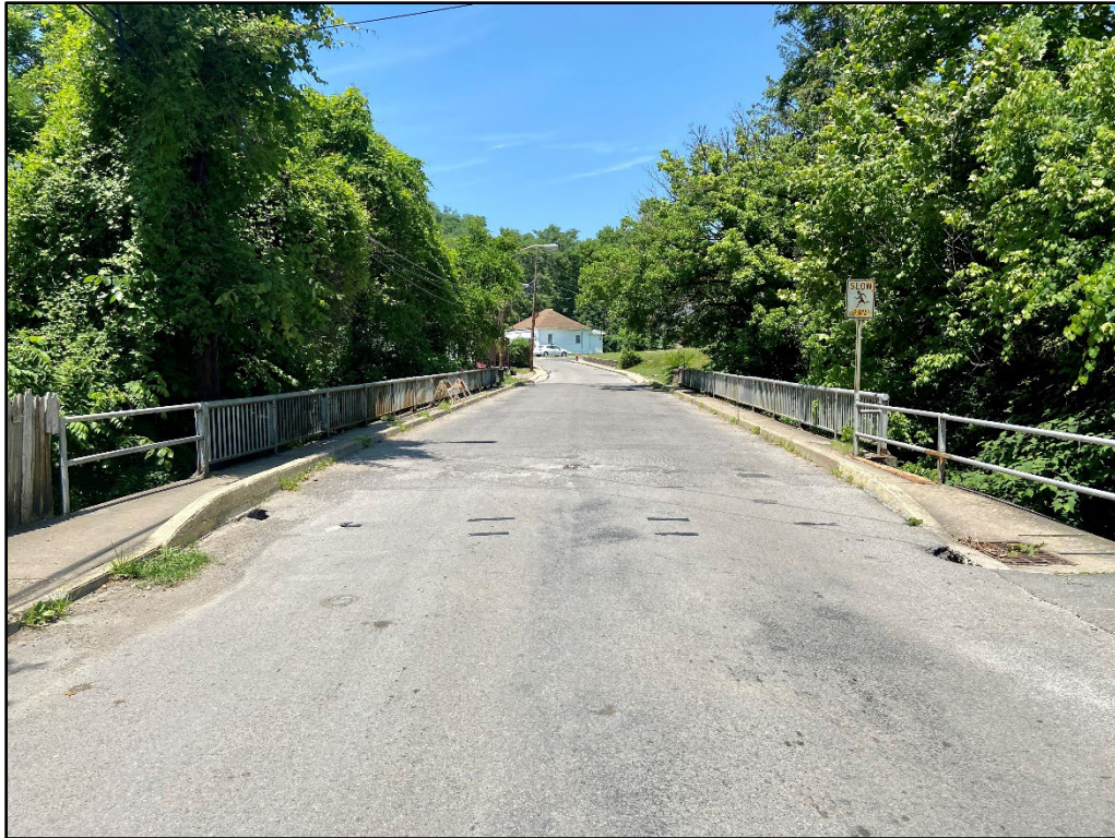
Photo 5: East Approach. View Northwest
