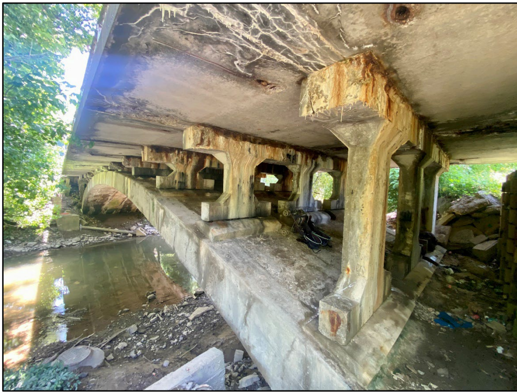
Photo 2: North (Upstream) Elevation. View South
