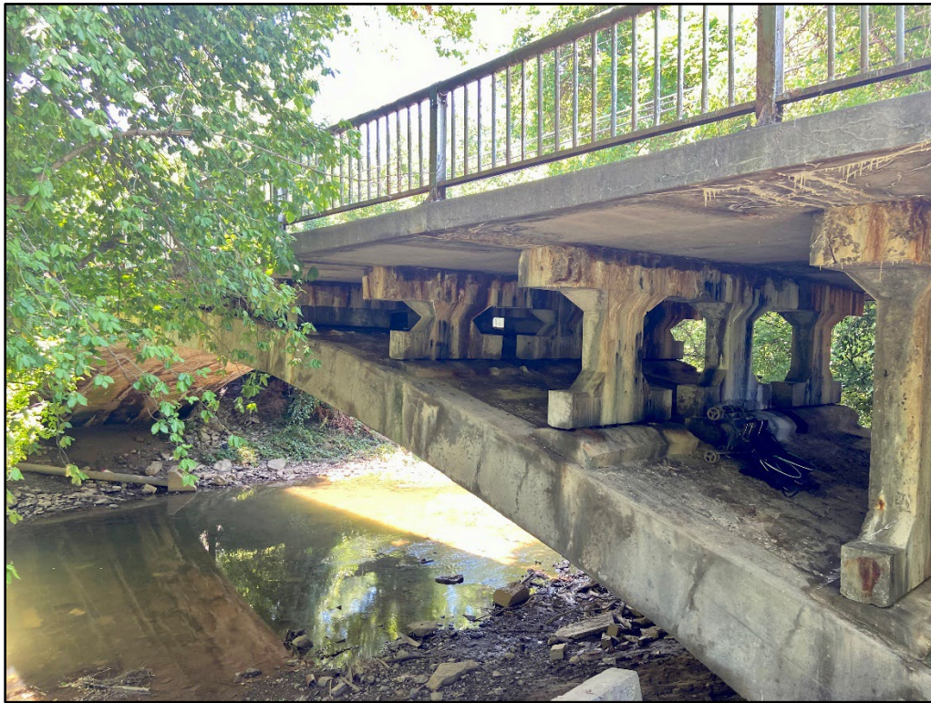
Photo 1: North (Upstream) Elevation. View South
