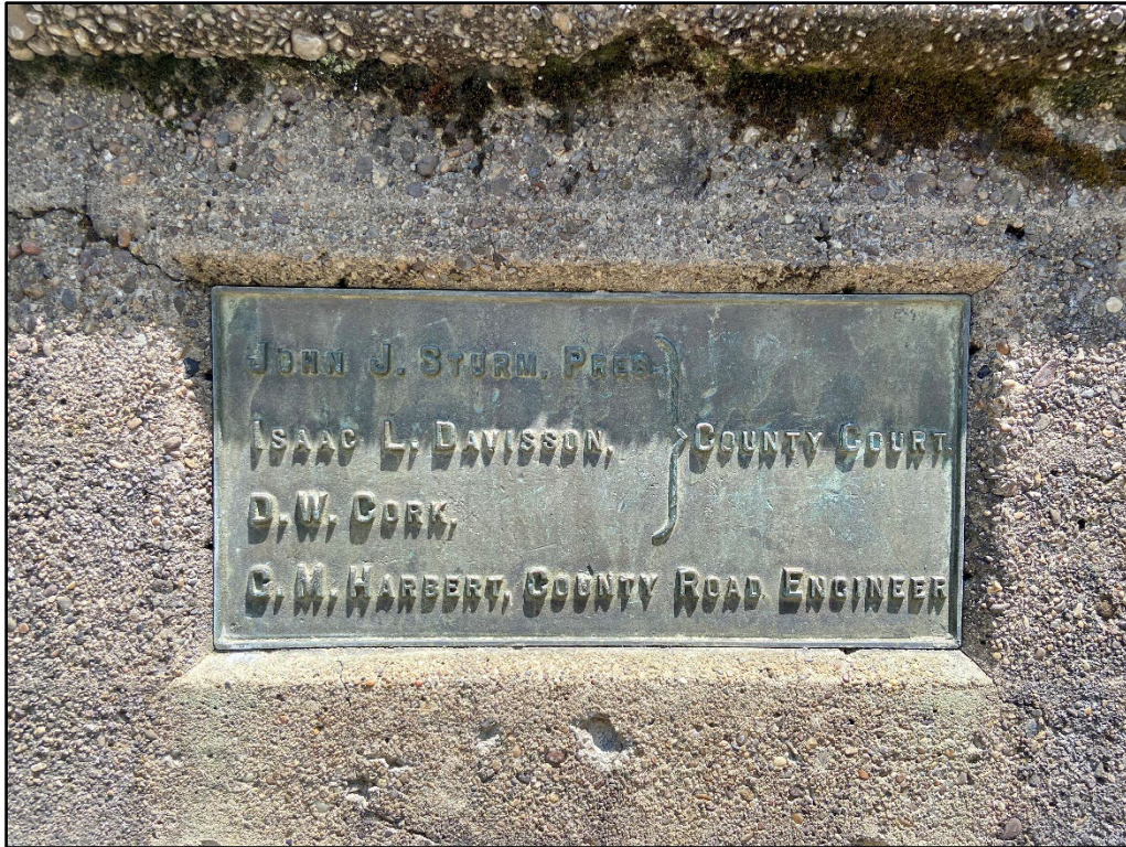
Photo 7: Metal Plaque at West End of North Railing. View Northeast
