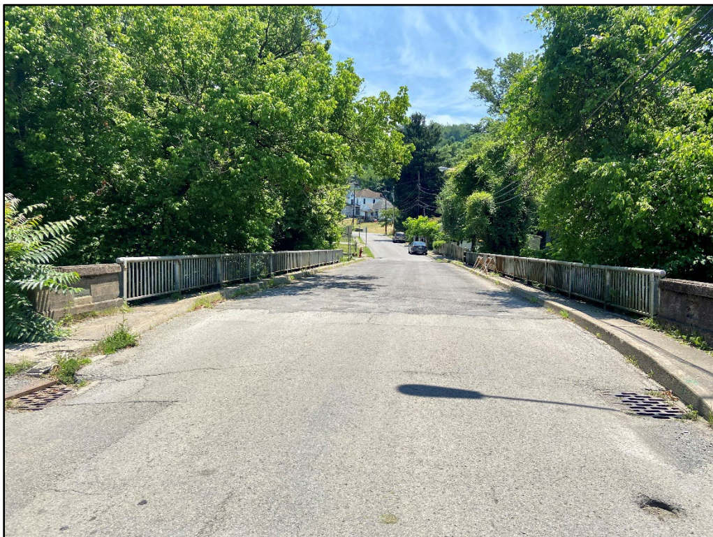
Photo 6: West Approach. View Southeast
