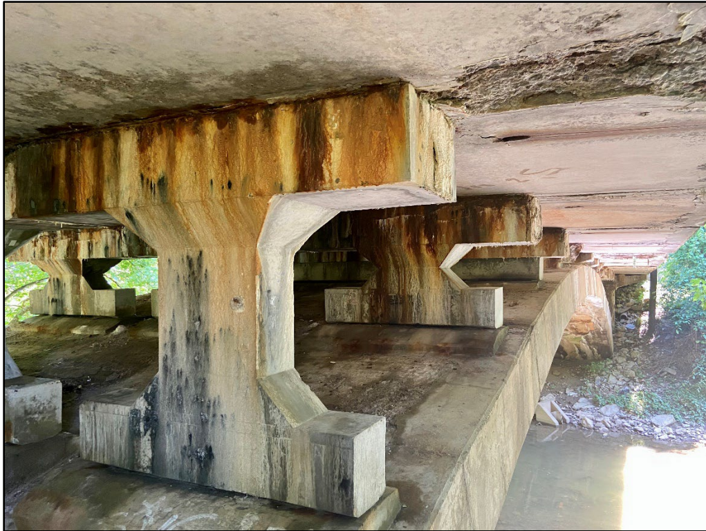
Photo 3: South (Downstream) Elevation. View Southeast
