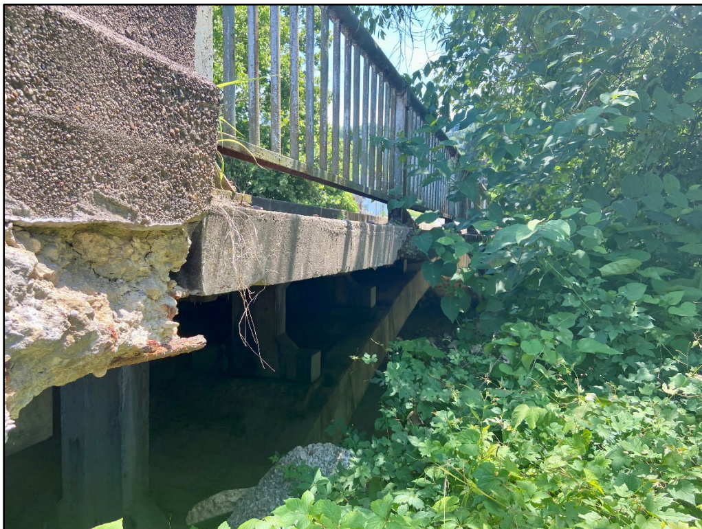
Photo 4: South (Downstream) Elevation. View Southeast
